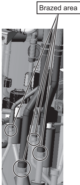
Removal of the rear heat exchanger on a high-efficiency model (Figure 15)
